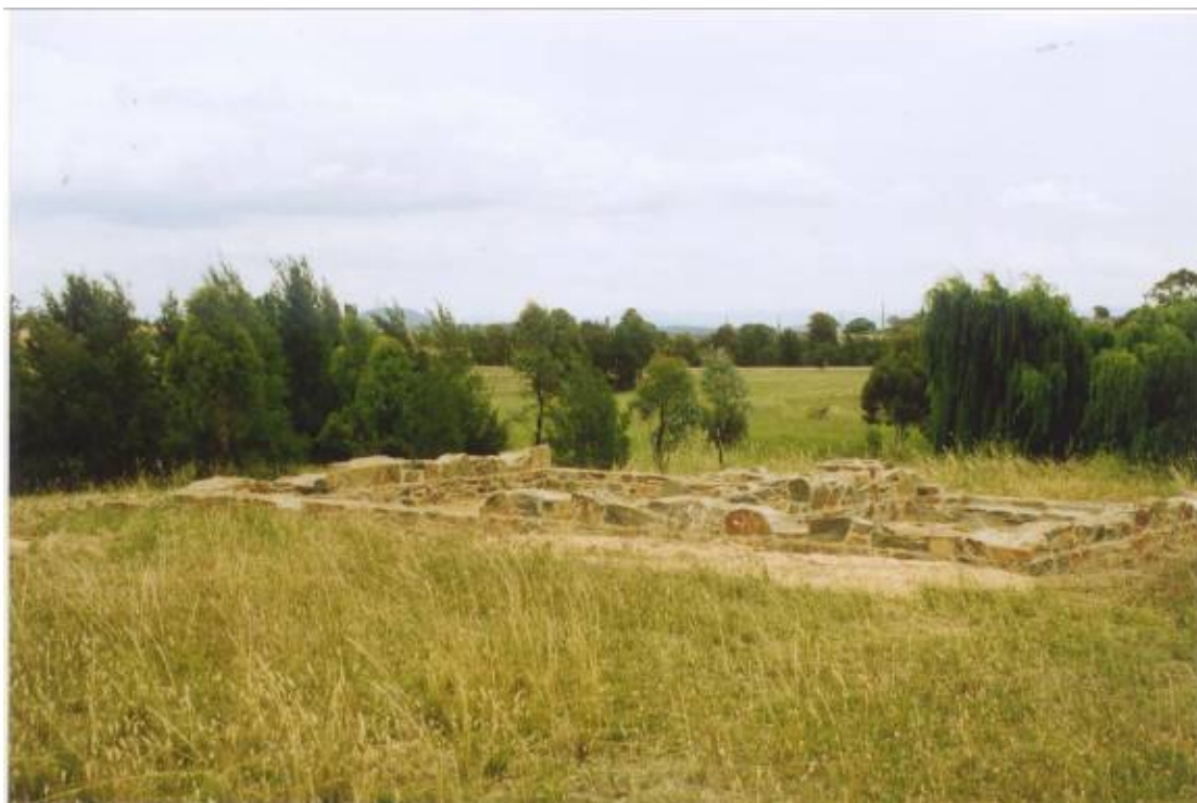
Crinigans Stone Hut site after stabilisation of the walls.
